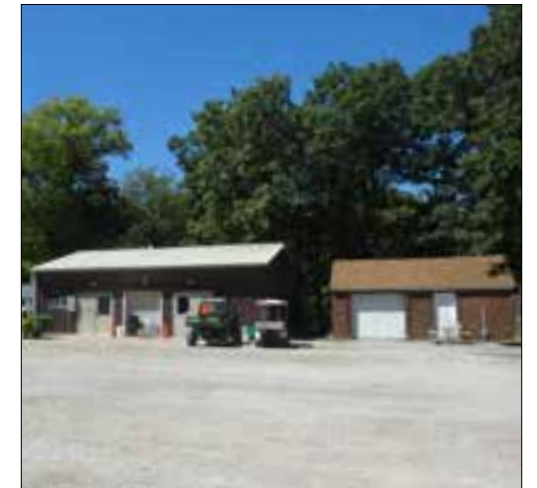
9 & 10. Commissary & Storage Building
