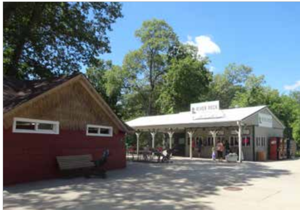
Existing restrooms and food to be replaced
